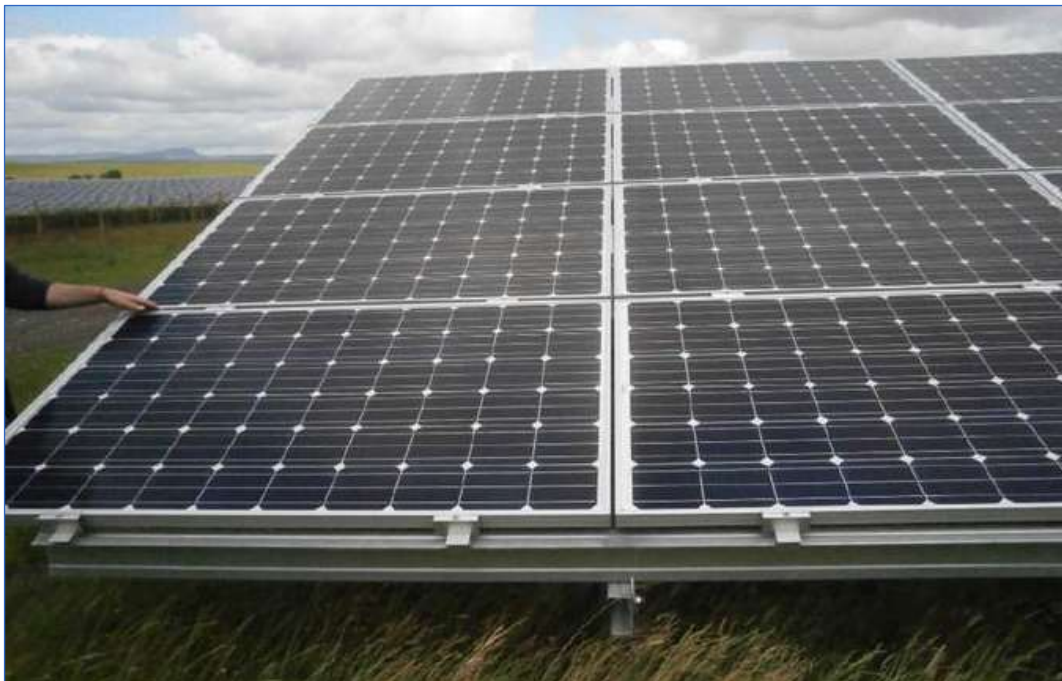
Figure 7-1 Typical Solar Panel Arrangement (showing expansion gaps)
